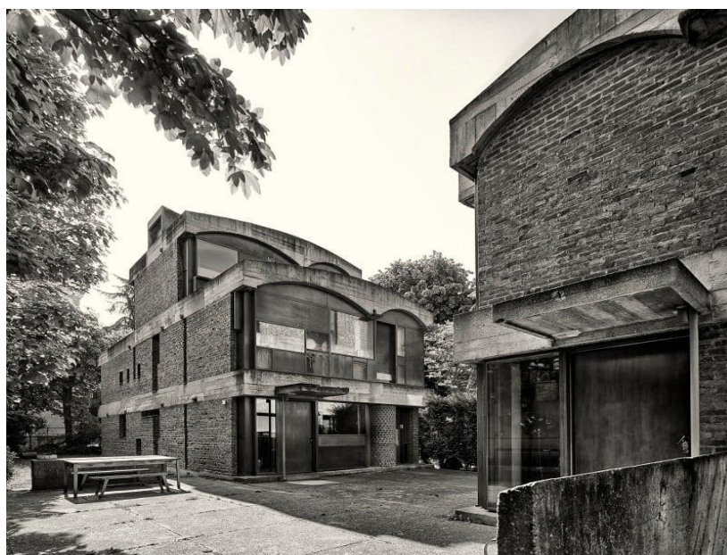
Figure 2 – Maison Jaoul (Photo of Cemal Emden)
