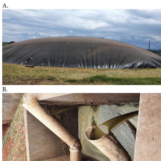
**Figure 1.** Anaerobic biodigester (A) and outlet pipe for inoculum biofertilizer (B)
