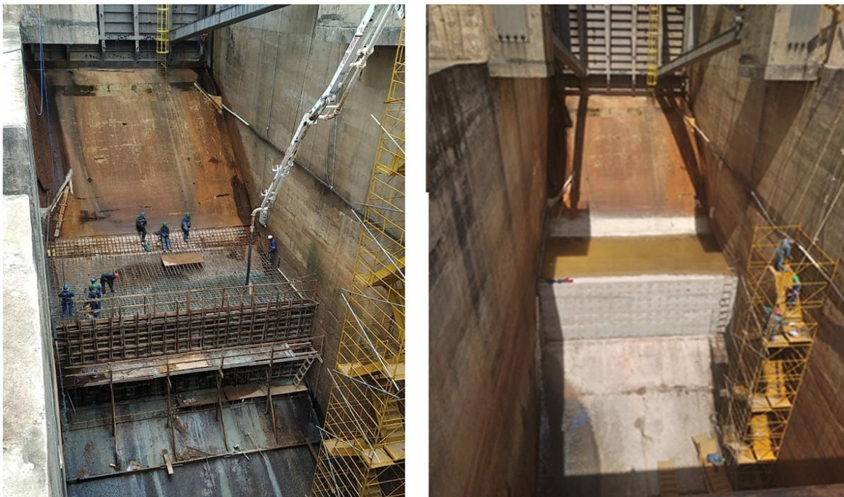
Figure 11. Deflector constructed into the spillway bay.
