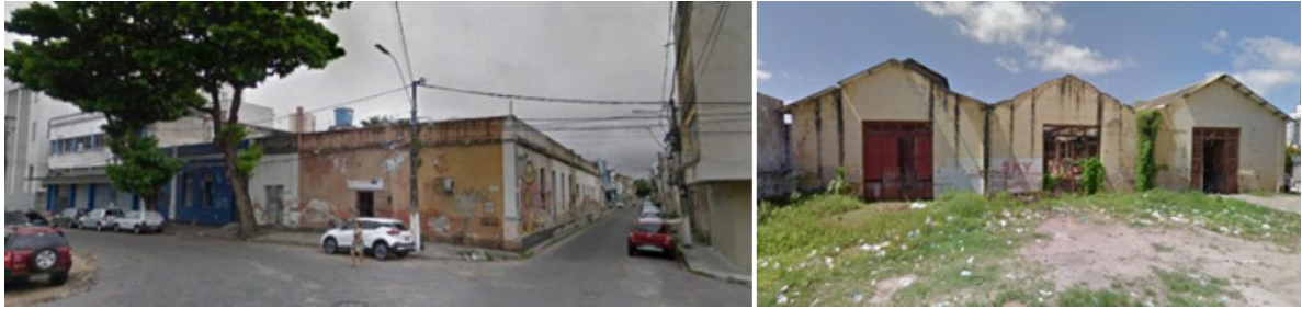
Figure 4 - SPU Building (left) and RFFSA Warehouses (right) requested by the MNPR for the construction of equipment and HIS to support the homeless population
