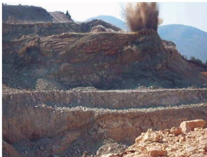
Figure 1 Drill cuttings are easily ejected from hole collar.
