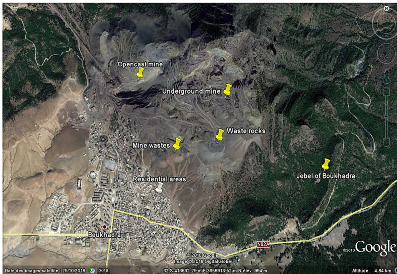
Figure 1 - General view on the mining wastes from the Boukhadra mine.
