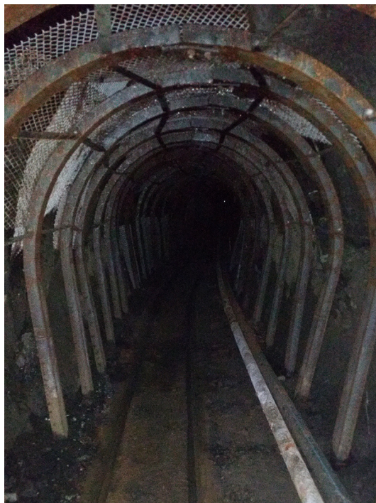
Figure 3 - Lateral ground thrust in gallery section.
