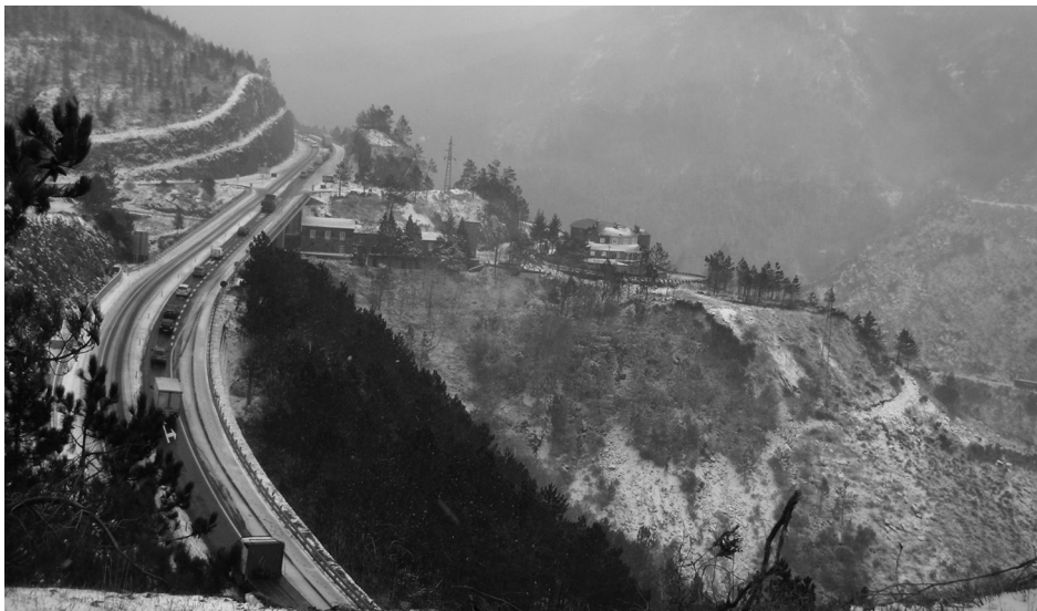
Figure 2 Highway A4 (author's photo).
