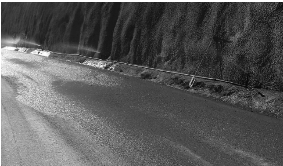
Figure 3 Humidifying system (author's photo).
