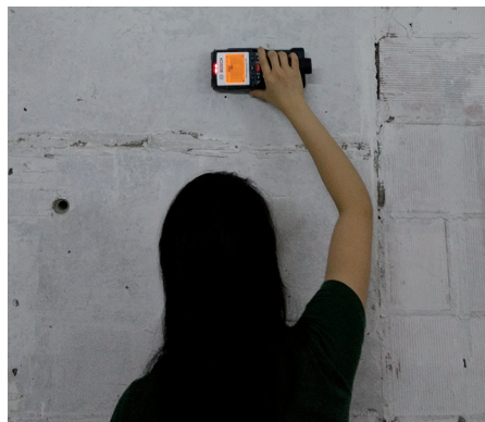
Figure 2 Placement of the pacometer on the column to detect the reinforcement.
