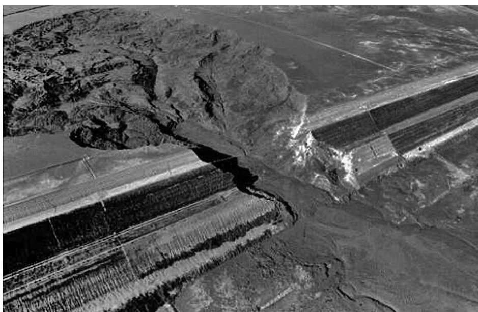
Figure 2 Rupture of the Marriespruit tailings dam in Virginia-South Africa, 1994. Source: Flood List (2018)
