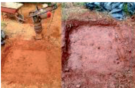
Figure 3 Sequence of compaction of the holes.
