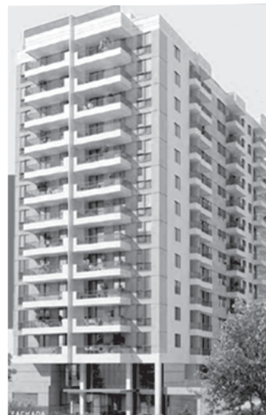
Figure 1 Building frontal view
