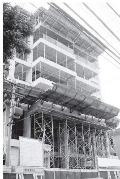
Figure 4 Construction aspect at the second construction stage
