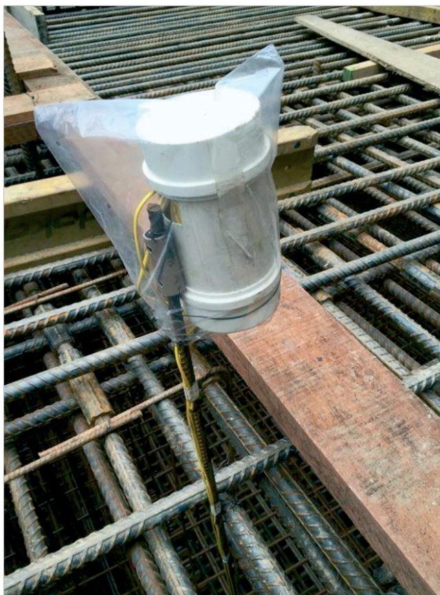
Figure 4 – Detail of thermocouple and data recorder attached to the footing reinforcement
