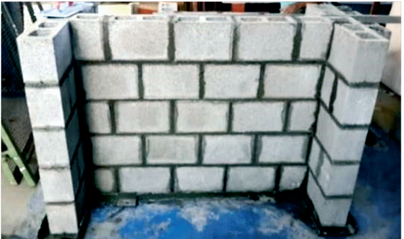
Figure 2 - Executed first step of the flanged wall
