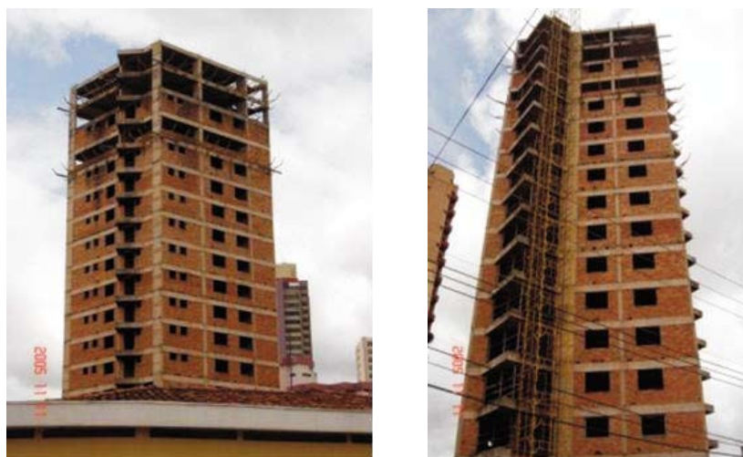
Figure 4 - Aspects of building "A"
