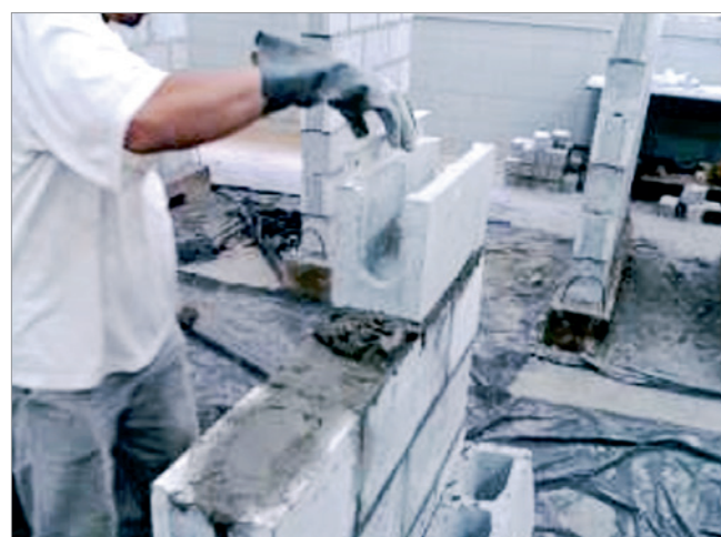
Figure 10 Mid-height bond beam laying
