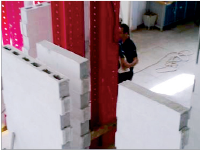
Figure 15 Walls capped with mortar
