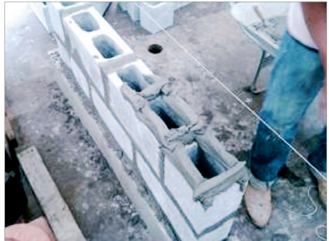
Figure 12 Full bed mortar joint wall construction
