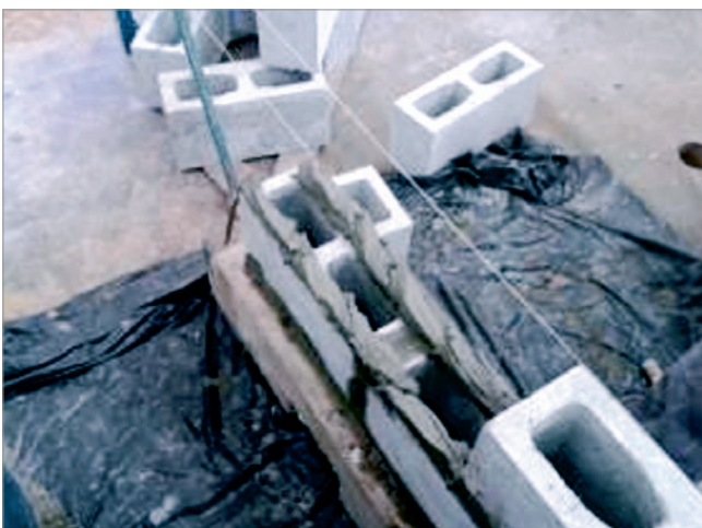
Figure 13 Face-shell bed mortar joint wall construction
