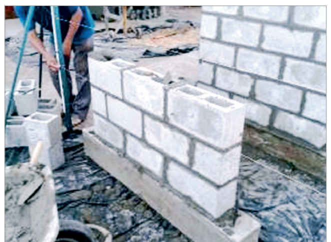
Figure 9 Hollow wall construction
