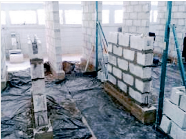
Figure 11 Wall with mid-height bond beam
