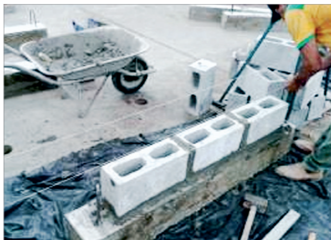
Figure 7 Corner gauge to aid wall construction
