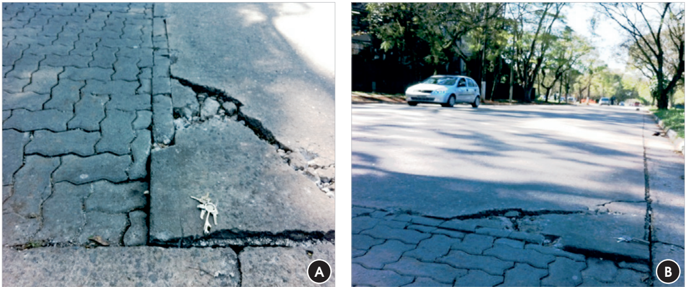
Figure 6 - Concrete deterioration at the transversal edge
