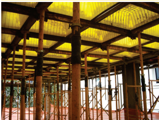
Figure 1 – Formwork developed for waffle slabs
