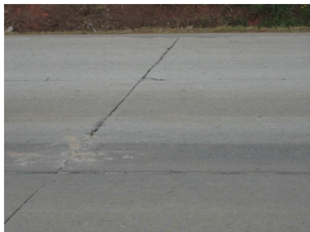
Figure 3. Concrete pavement prior to removal.
