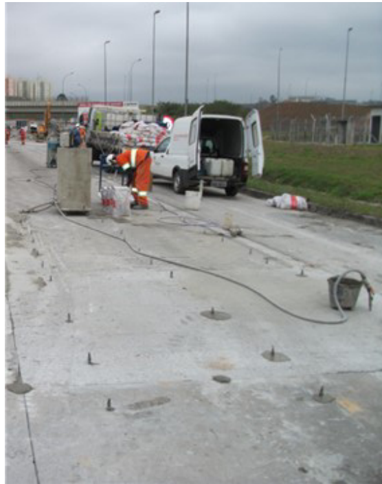
Figure 2. Cement slurry injection at KM 30 in 2011.
