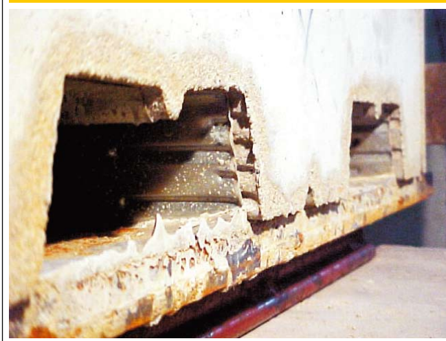
Figure 7 - Series A - Prototype 2 - Observed end slip at ultimate applied load
