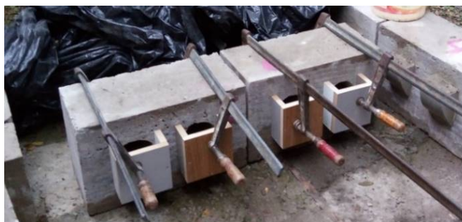
Figure 2 – Molds for concrete and grout repair
