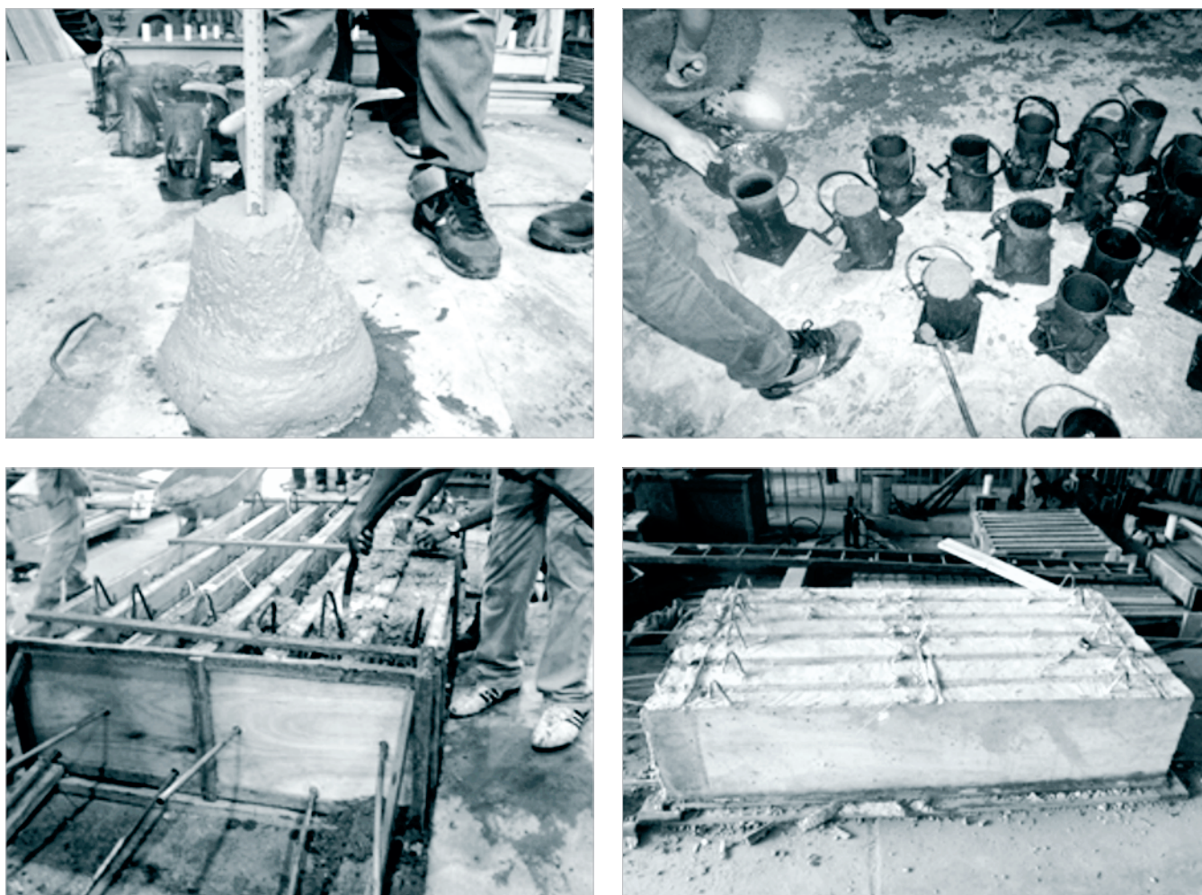
Figure 5 - Beams' executive process
