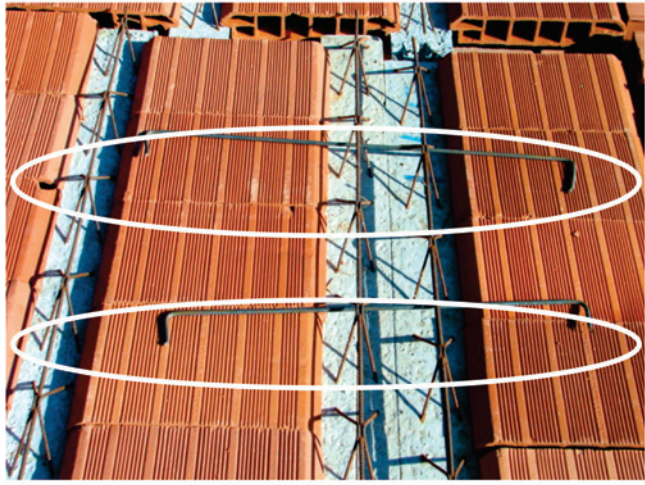
Figure 9 – Negative moment rebars
