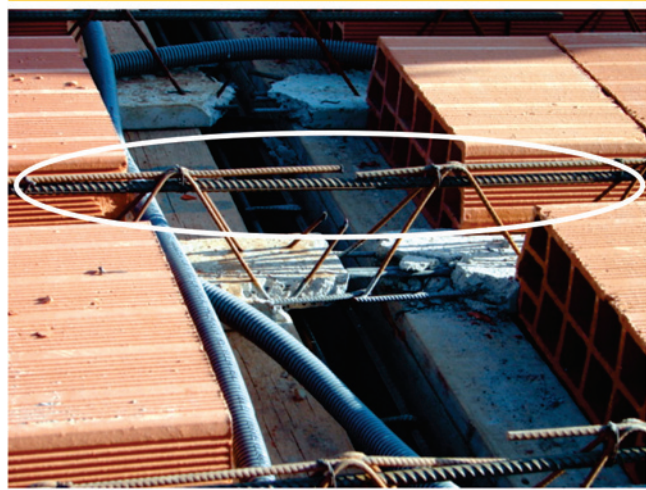
Figure 6 - Negative moment continuity rebar
