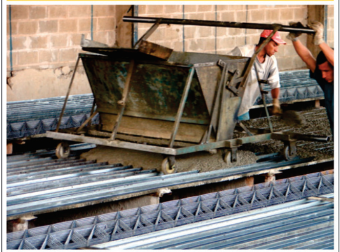
Figure 3 - Concrete poured using a mechanism created by the manufacturer
