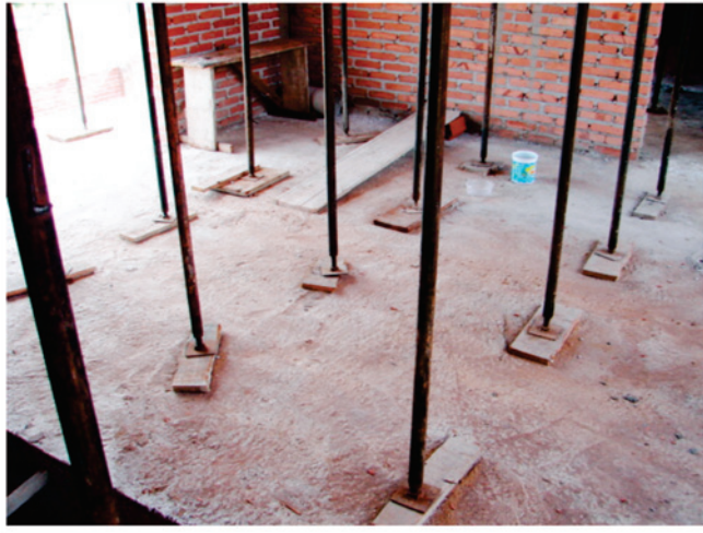
Figure 11 – Falsework bars supported on boards
