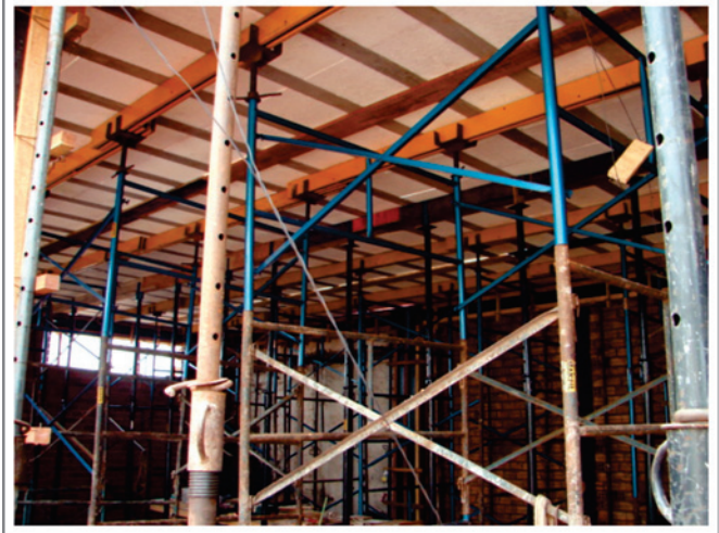
Figure 10 – Falsework system
