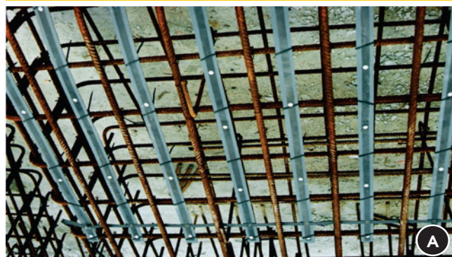
Figure 7 – Tapes installation (a). Concreting (b) Electric power supply (c). General view after repairing (d)
