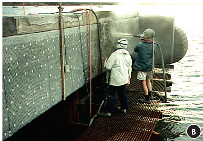
Figure 4 – Activated titanium mesh application. Mesh fixation on the concrete surface (a). Cover mortar applied by projection (b)
