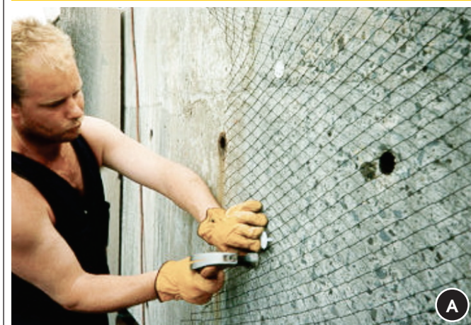
Figure 4 – Activated titanium mesh application. Mesh fixation on the concrete surface (a). Cover mortar applied by projection (b)
