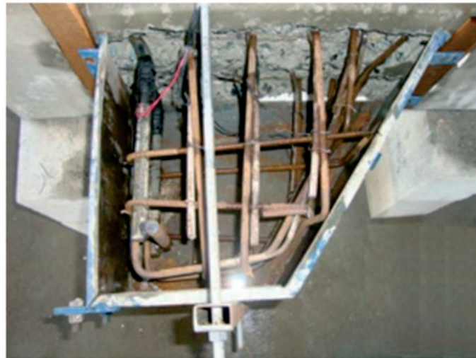
(c) Column-corbelt interface after scarification and reinforcement turned to straight and ready for casting of the corbel (models P3, P4, and P5)
