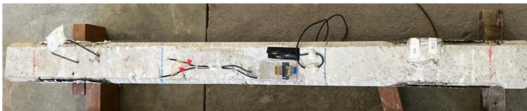
Figure 9. View of the sensors on one of the beams.
