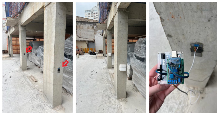
(a) Plates installed (b) Protecting the plates (c) Data system connected
