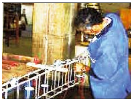
Longitudinal reinforcement placement
