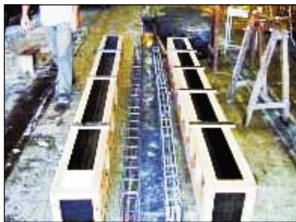
Frameworks and reinforcement cages
