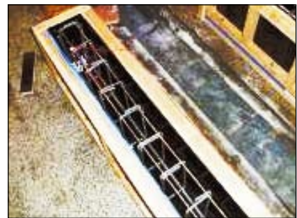
Beam ready to be cast
