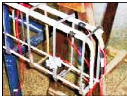
Placement of steel stirrups
