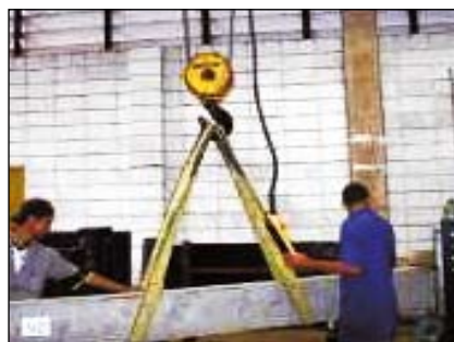
Transport of the beam
