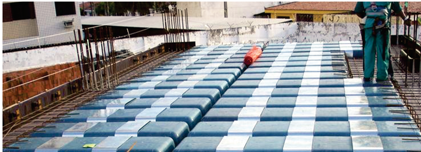
Figure 3 – One-way waffle slab, OWWS
