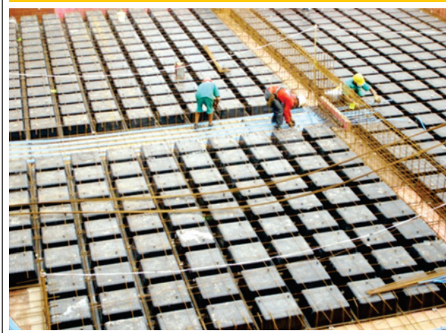
Figure 2 - Two-way waffle slab, TWWS
