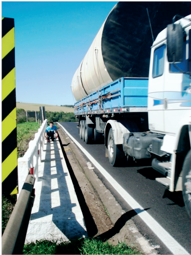
Figure 6 – Source of vibration of the structure for a sample on viaduct V1
