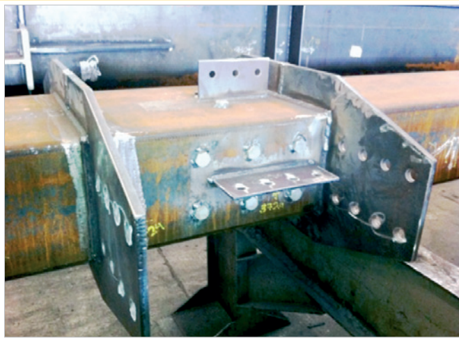
A Join with steel plate welded
