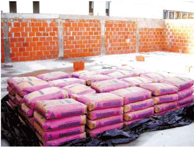
Figure 17 – Structure totally loaded
