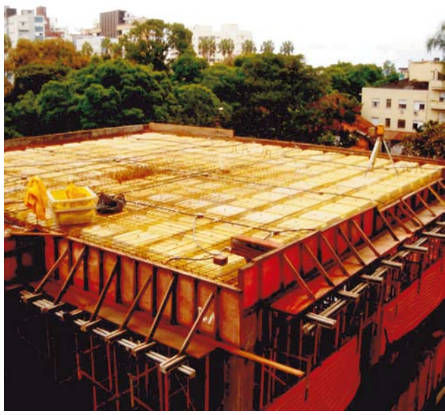
Figure 13 – Slab before casting
