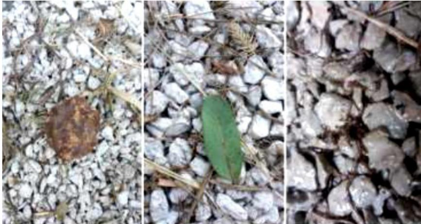
**Figure 4.** Debris over sidewalk porous concrete surface: dry leaf (left); green leaf (center); rotting organic matter in between aggregates (right).
