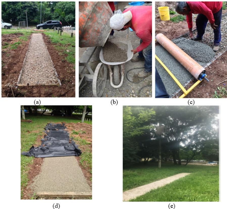
**Figure 5.** (a) Recycled aggregates sidewalk base and lateral metallic forms for concrete pouring; (b) in situ concrete provision with small concrete-mixer; (c) Concrete pouring and compaction with light roll; (d) concrete curing using polyethylene fabric (7 days); (e) Final pervious concrete sidewalk view (December 2015).
