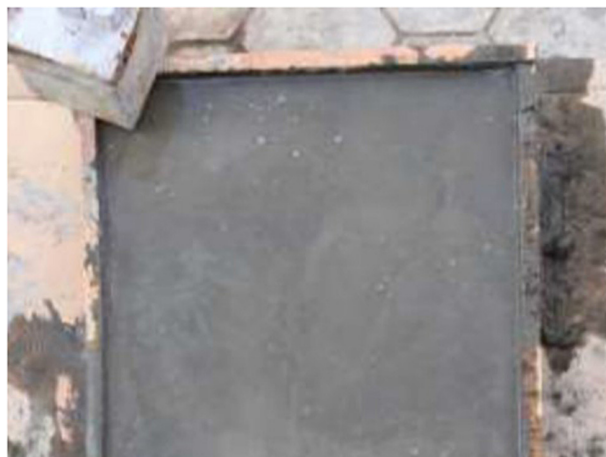
Figure 7: Slab concreting – bamboo reinforced concrete slab.
