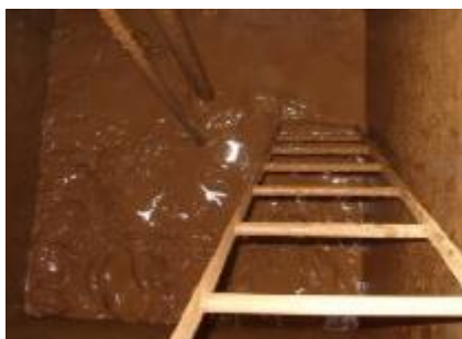
Figure 3: WTP sludge in the thickening tank.
