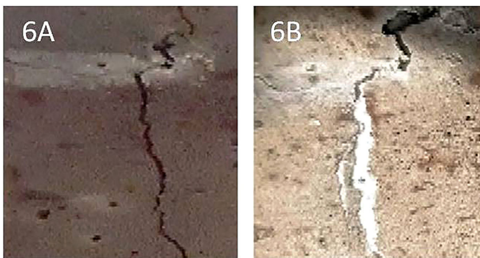
Figure 6: (a), (b) Crack image before and after healing of crack in specimen with bacillus flexus .
