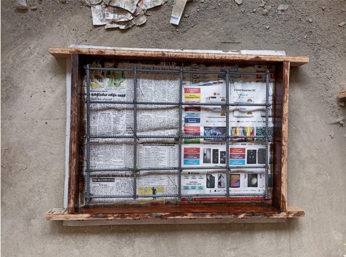
Figure 1: Placing of reinforcement.
