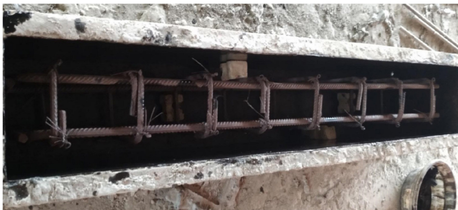
Figure 3: Placing of reinforcement in the mould.
