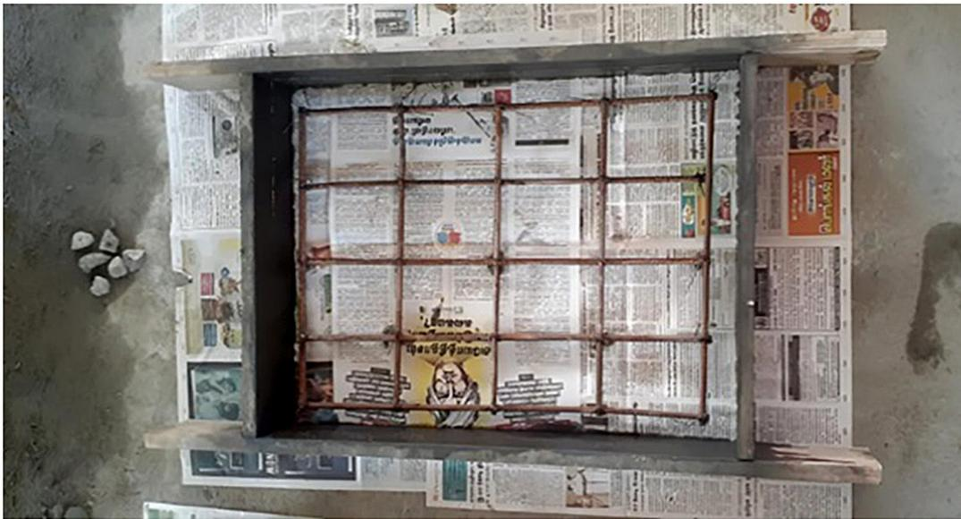
**Figure 3:** Placing of reinforcement.
