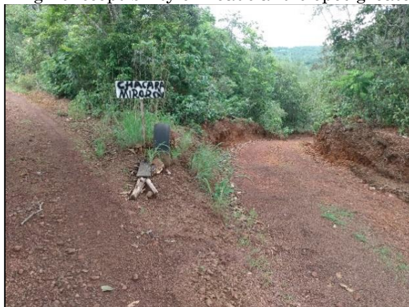
Figure 10 – High susceptibility on roads and slopes greater than 15%.
