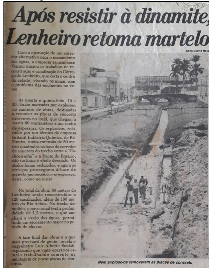
Figure 10 – Demolition of the canalization
