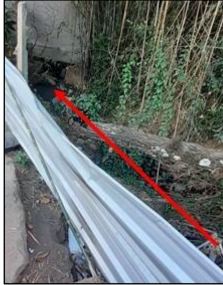
Figure 20 – House over the Caieira stream
