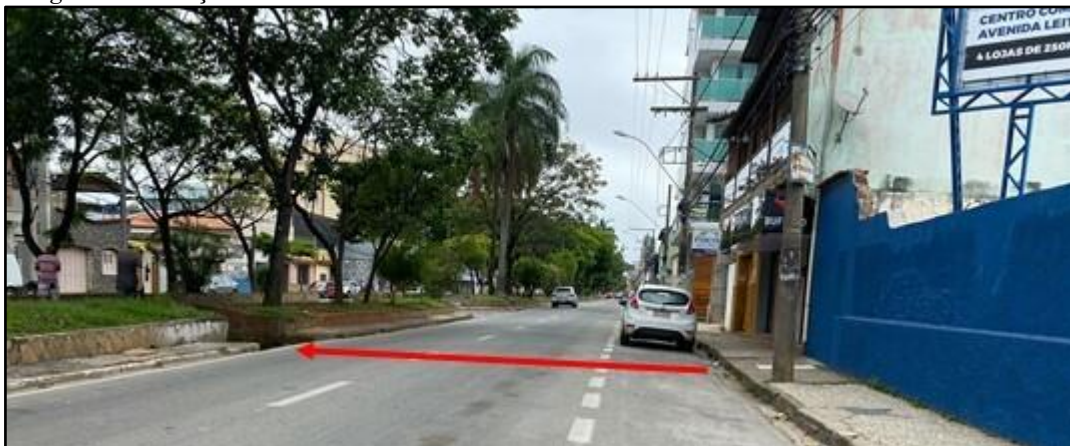
Figure 22 –Voçoroca do Dom Bosco stream canalized under Leite de Castro Avenue
