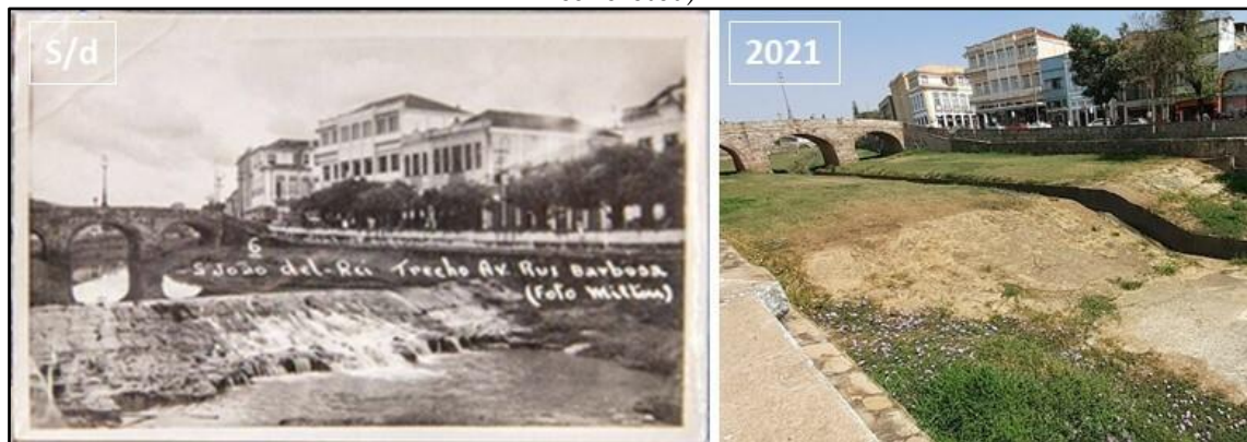
Figure 3 – Falls of the Lenheiro stream (natural in the black and white photograph and currently concreted)
