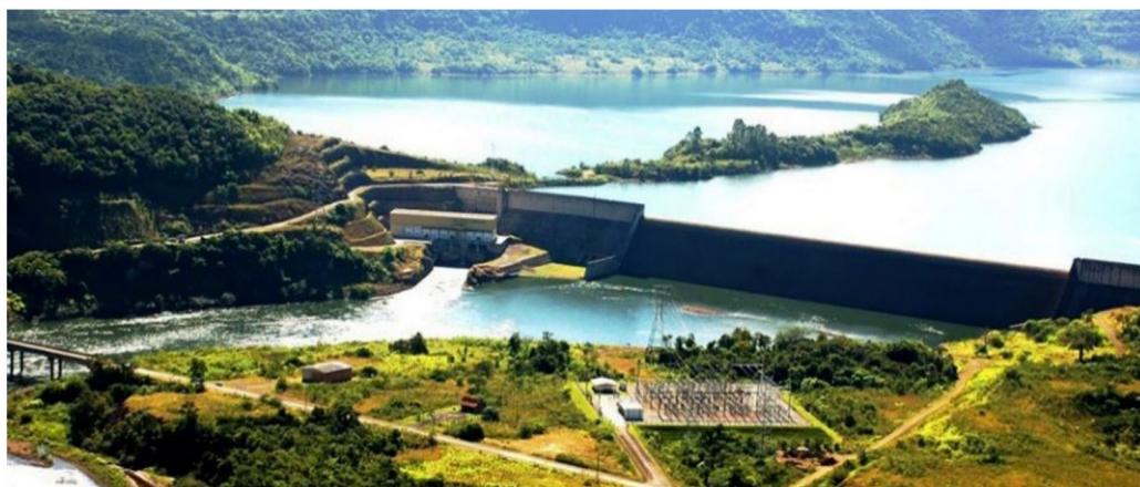
Figure 1. Panoramic view of the Dona Francisca dam.
