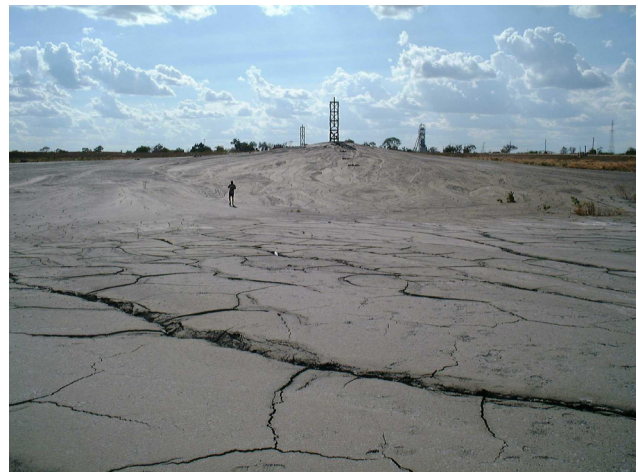
Figure 2. A thickened tailings site, where a relatively fresh layer can be distinguished from the underlying desiccated layer (Courtesy Jason Crowder).
