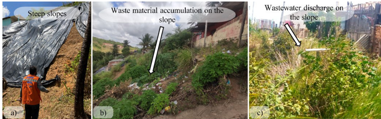
Figure 2. Scenarios identified in the study areas: a) steep slopes; b) waste material accumulation on the slopes; c) wastewater discharge on the slope.
