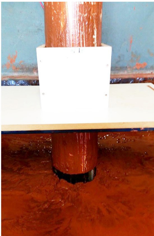
Figure 2. Installation of the column using a wooden casing.
