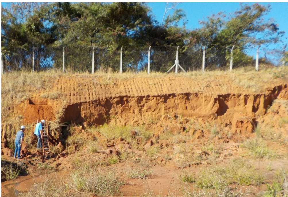
Figure 13. The slope after failure [adapted from Vieira (2021)].
