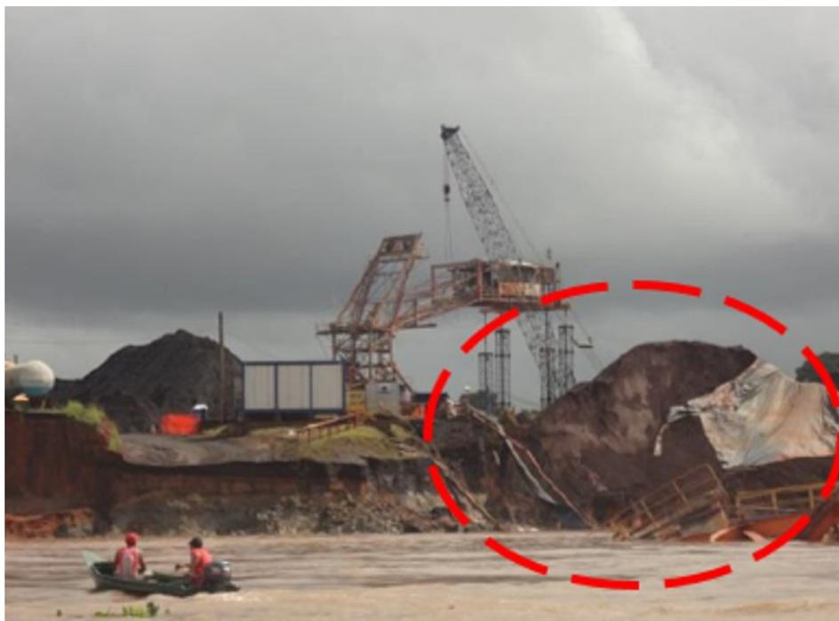
**Figure 5.** View of the post-failure scenario, highlight for the remaining stockpile, East side (modified from Brazil, 2014).
