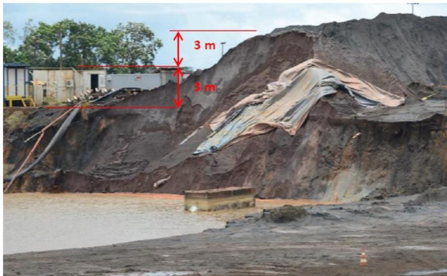
**Figure 7.** Detail of the remaining stockpile at the eastern side, indicating that the failure occurred for a stack height of 6 m (Pacheco et al., 2014).
