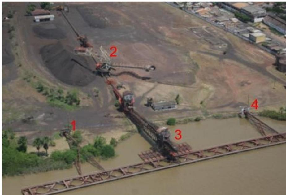
**Figure 2.** Scenario of the 1993 failure: 1) west truss; 2) stack reclaimer; 3) conveyor belt; and 4) east truss (Pacheco et al., 2014).
