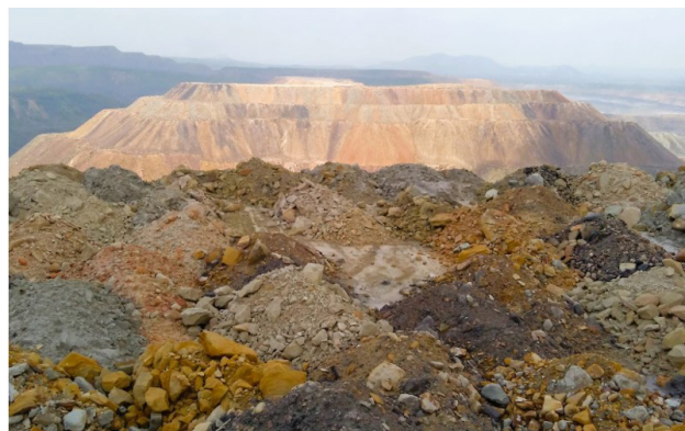
Figure 3. View of different materials with varying particle sizes that contribute to the formation of a dump.
