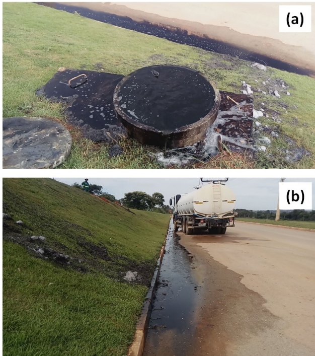
Figure 4. Leachate leaks: (a) gas drainage with leachate; (b) flow of leachate along the road.
