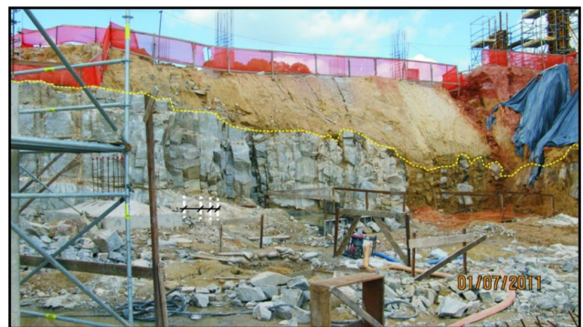
Figure 3. Aspect of slope of Southeast Sector.
