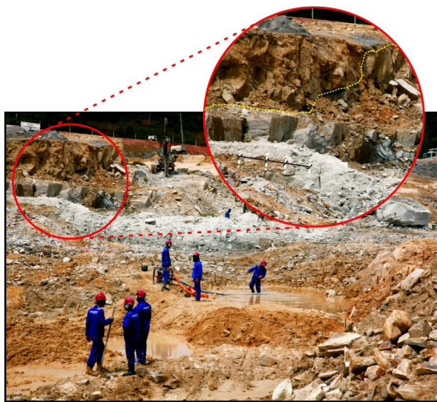
Figure 4. South Sector with occurrence of boulders on its surface, zones of weathered and fractured rock.
