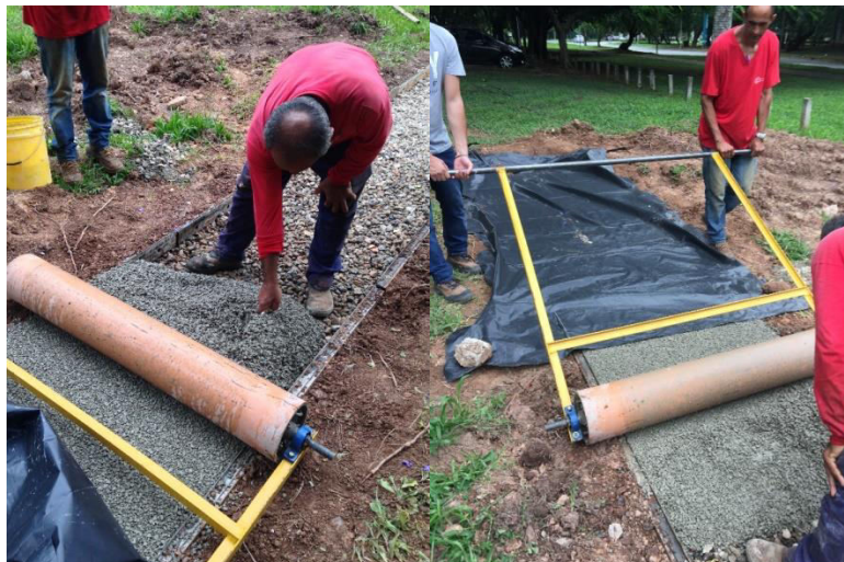
Figure 3 - Pervious concrete laying for the sidewalk slab test
